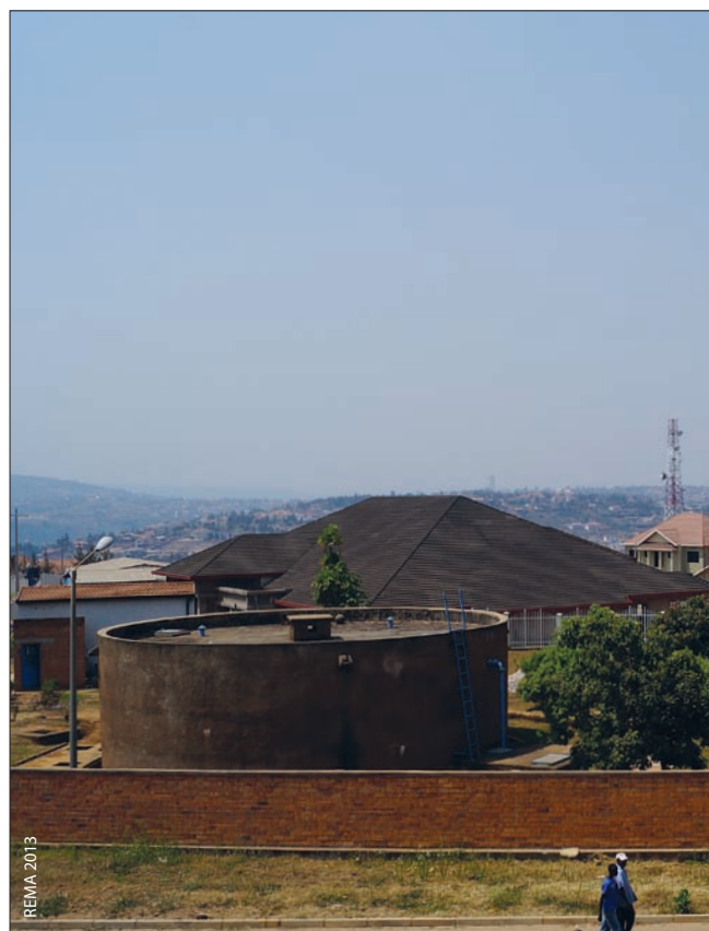
Water storage tanks supplying the Gacuriro neighbourhood
