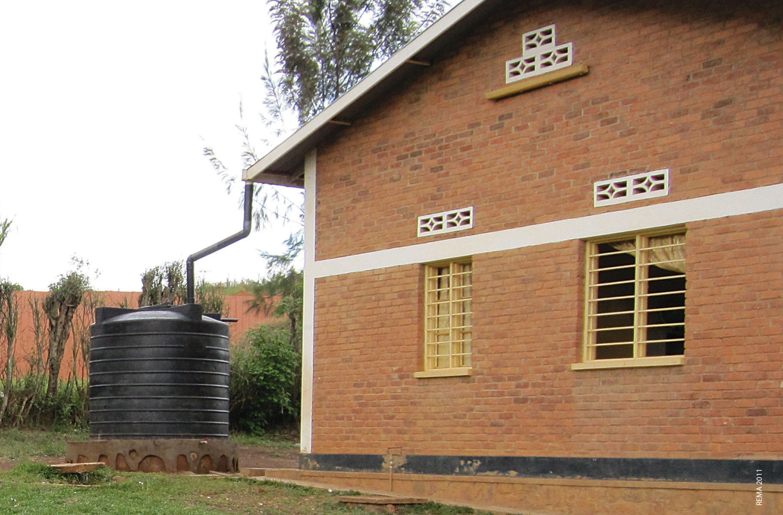
Rainwater harvesting from a school roof is being used to establish and maintain a playground lawn
