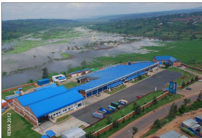
Heavy flooding (shown in this photo; taken after floods in May 2012) caused stagnant water to accumulate near the Inyange Industries and contributed to damage of infrastructure
