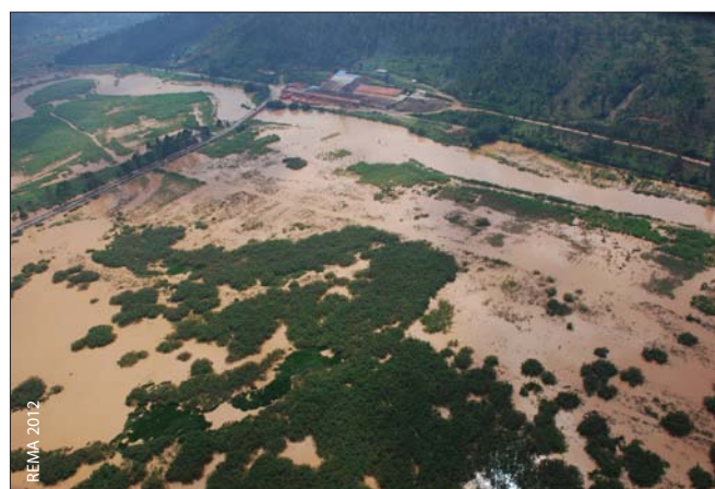
Flooding at Ruliba Clays
